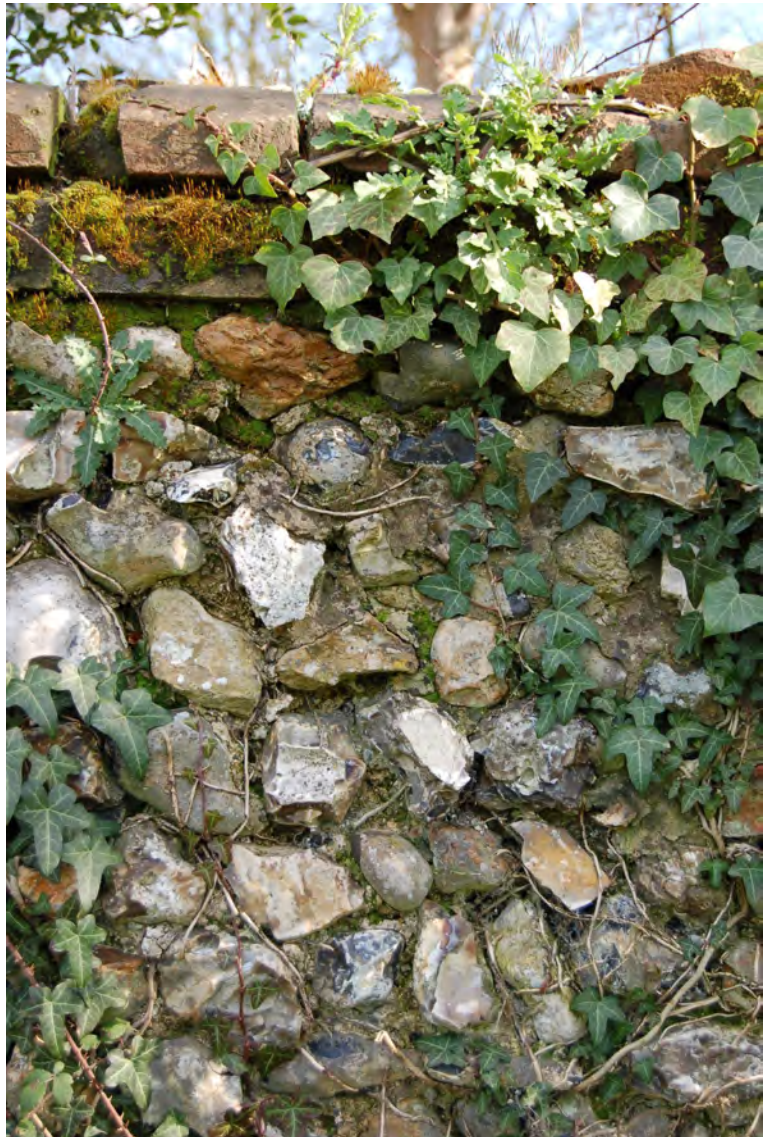
Picture 2.3 Quality flint wall with half round brick cap adjacent to St Mary's Church
