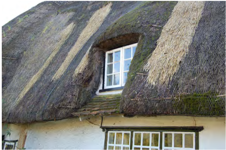
Picture 2.1 Low thatched dormer with tiled run-off detail to a property in The Row
