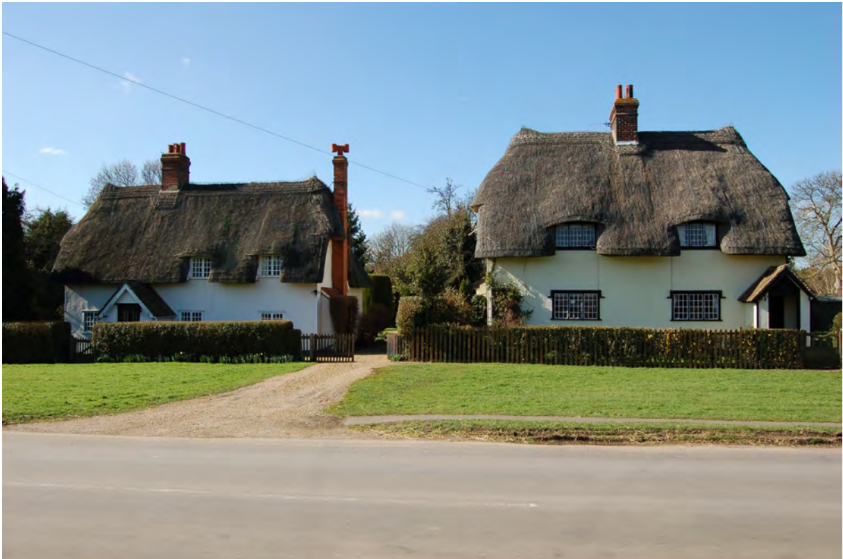
Picture 1.22 Suckling Cottage and Cedar Cottage, two quality listed buildings on Crow Street
