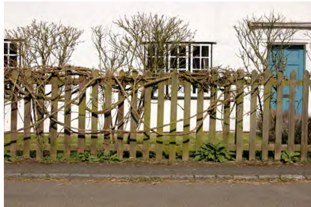
Picture 1.10 Timber fence to the front of Mount House, Church Street. This style of fencing has been in use in this location for at least a century
