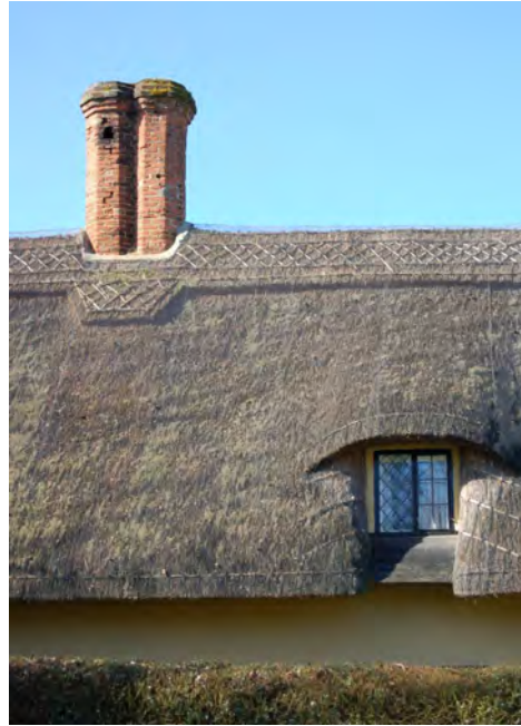
Picture 1.9 Thatched roof, narrow window aperture and quality chimney in Church Street
