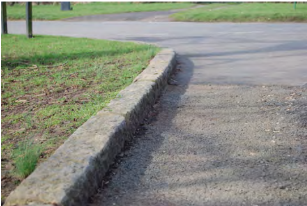
Picture 1.31 Quality granite kerb stones demark the edge of the green
